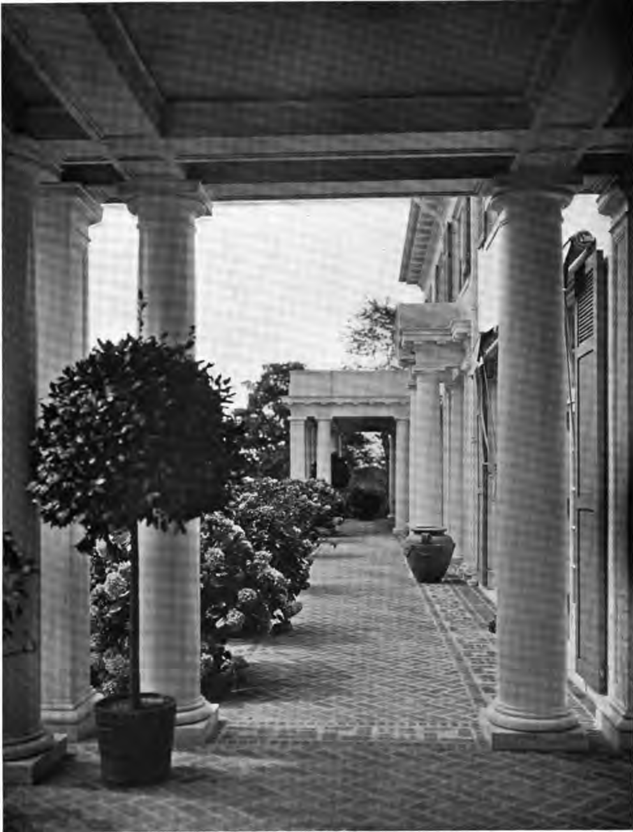
RESIDENCE OF DR. ERNEST FAHNESTOCK, SHREWSBURY, N. J. ALBRO & LINDBERG, Architects
