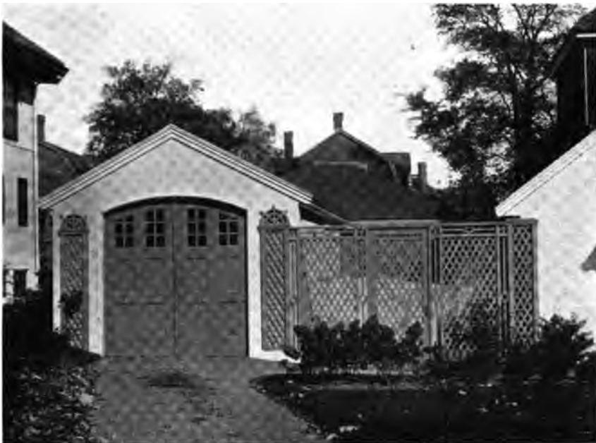
GARAGE AND FLOOR PLANS OF RESIDENCE OF MR. W. M. LIBBY, LYNN BOULEVARD, LYNN, MASS.
